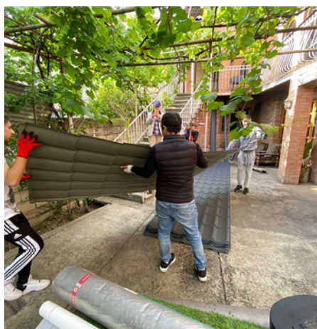
Roof renewal at NGO Mkurnali, Tbilisi
